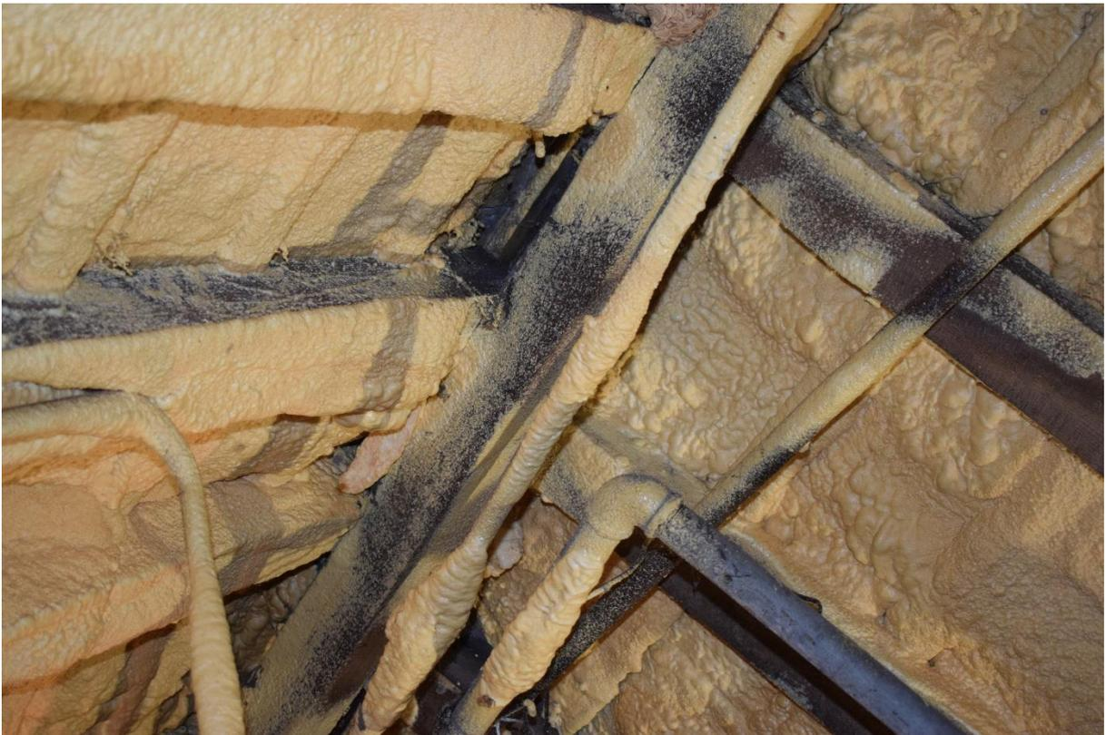
**Image: Tile stabilising closed cell spray foam**
