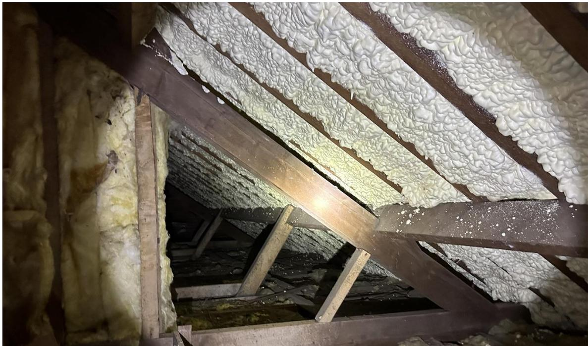
Image: Insulating open cell spray foam
